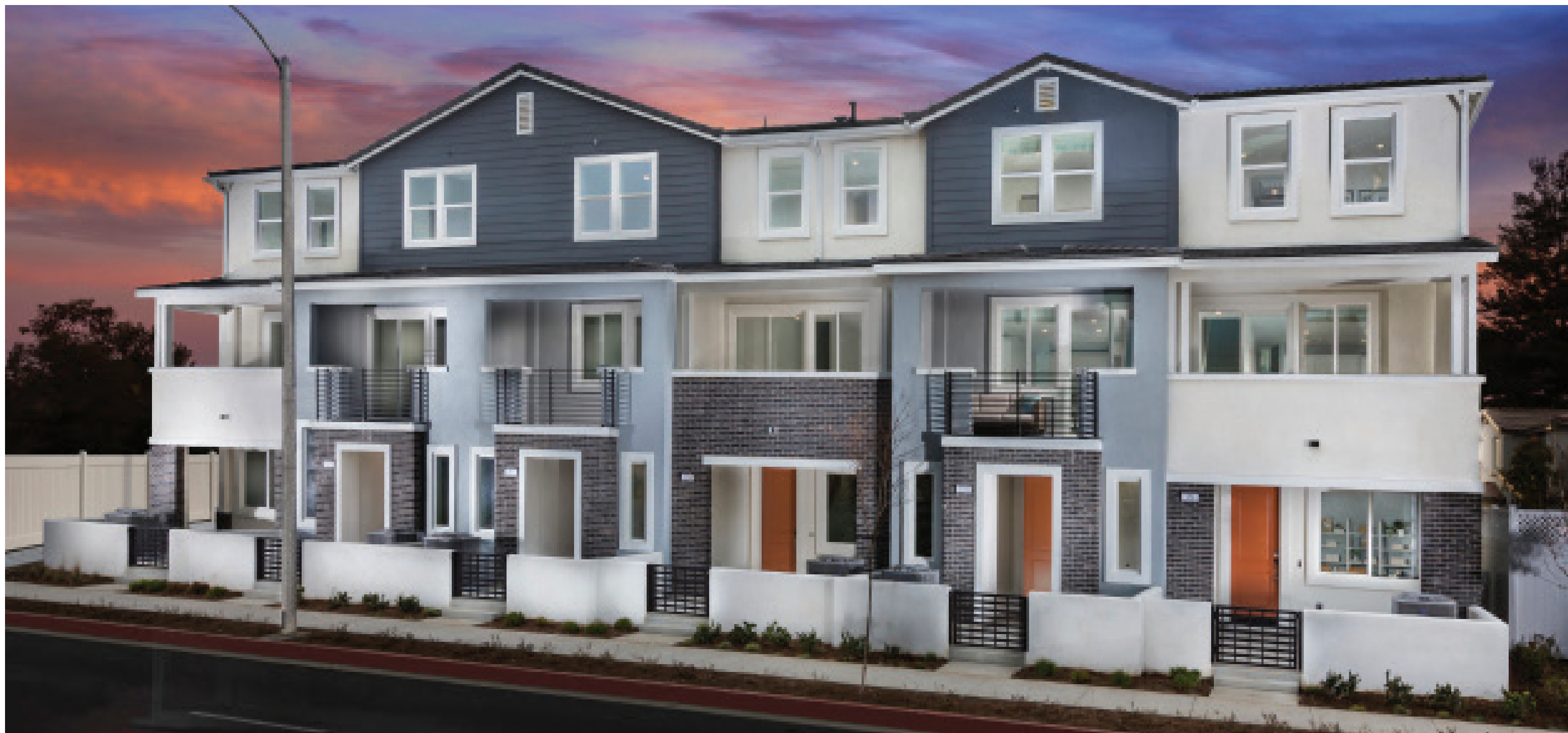
Seville at Vincent Place, West Covina
