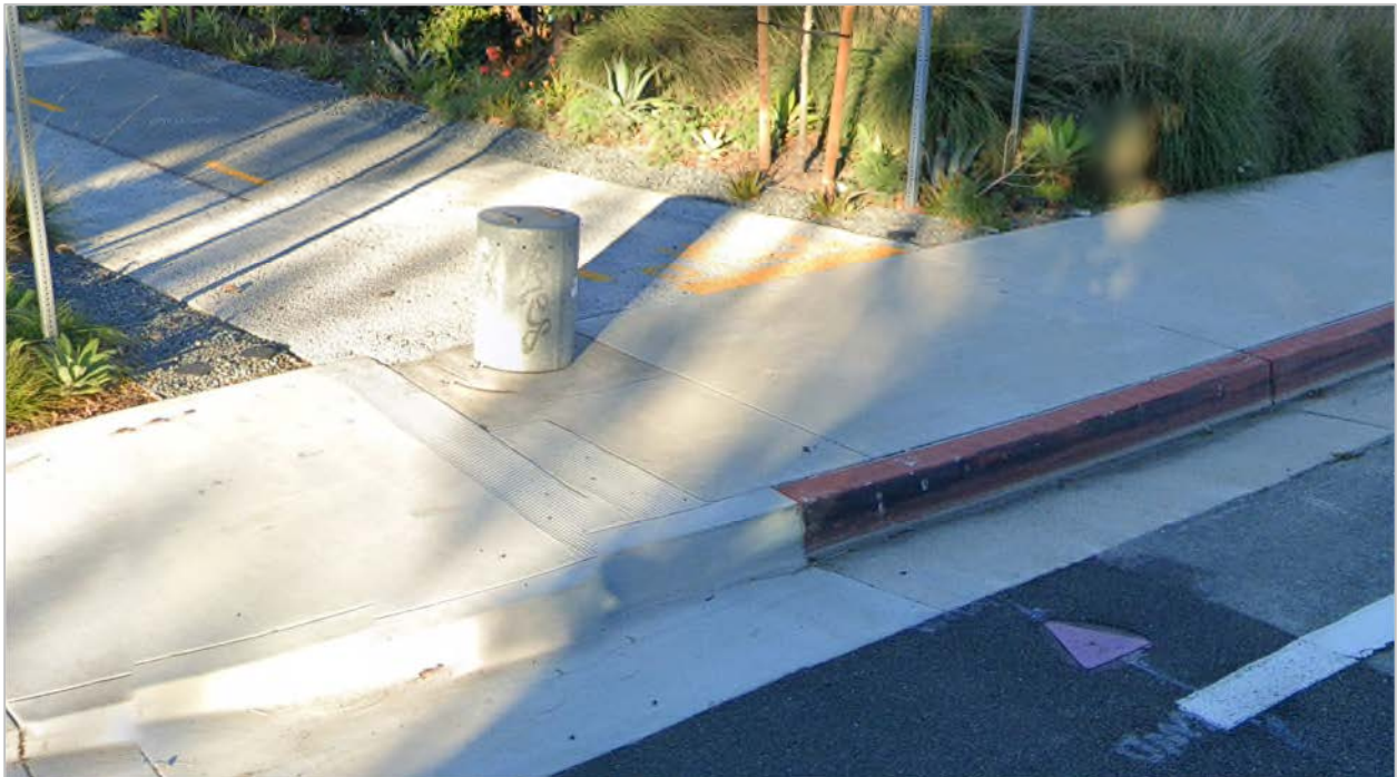
Figure 6. Existing Recycled Water Infrastructure
