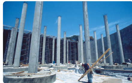
Reservoir 1 Construction in 1988
