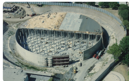
Reservoir 2 Construction in 1992
