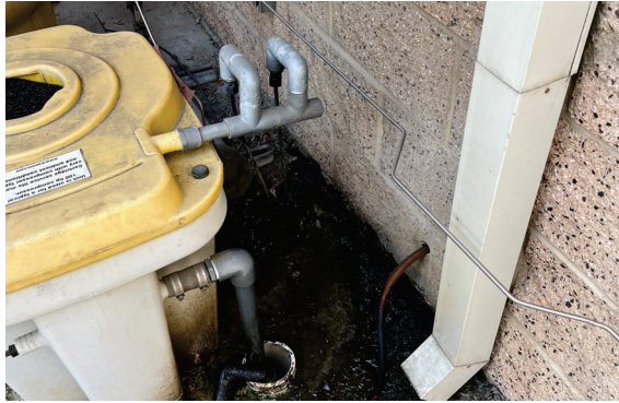
Quarterly Facility Inspection Checklist (IIPP)
